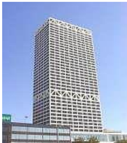
First Wisconsin Center, Milwaukee, USA
